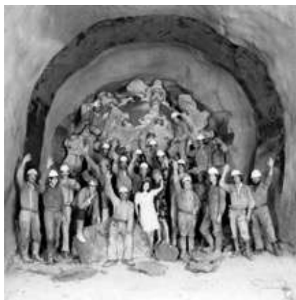
Proton Super synchrotron tunnel, 1974
