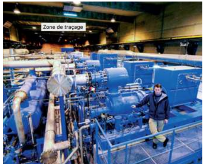
One of the 8 groups of refrigeration compressors used by the current LHC (Image: CERN)
